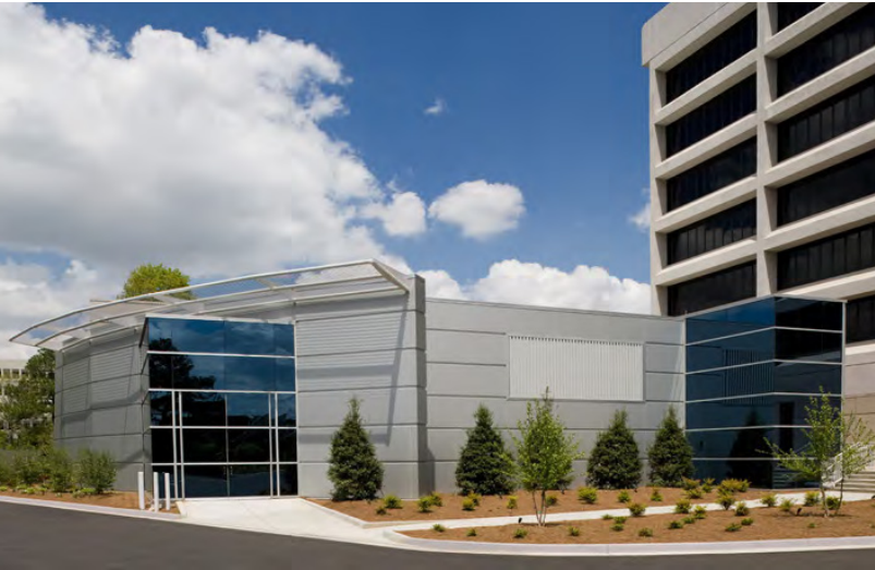
Weather Channel Studio and Data Center Expansion, Atlanta, Georgia, United States
